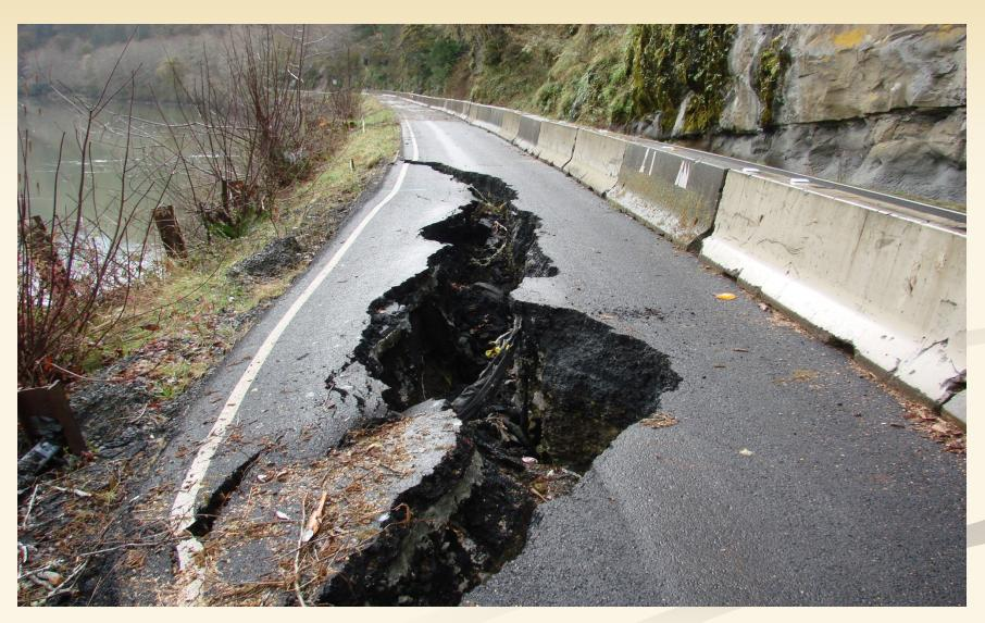
Damage to the road due to retaining wall failure. 10 years of progressive deterioration. Major funding through Grants. Project completed 2013.
